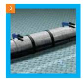
Use rubber band to fix the galvanized iron sheet andnail the sheet outer edge.
