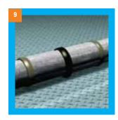
After 1 minute of foaming,cut the spilled foam and place a piece of galvanized iron sheet or moisture-proof tape on top of the hole.
