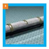
When the PU foam is about to reach the top of the hole, apply the rubber tape gently to cover the hole and let a little bit of foam leak out in order to squeeze out the air.
