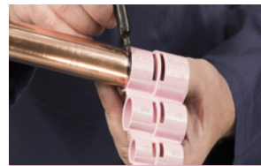
7a. Mark insertion depth on tube using depth gauge
